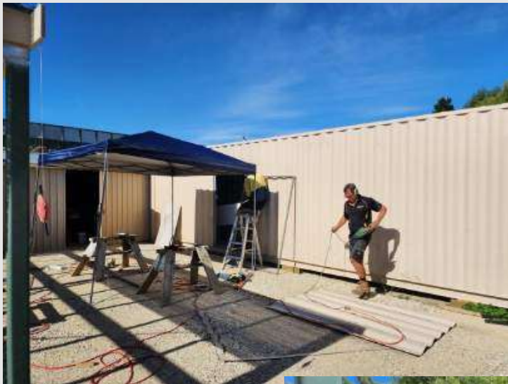
The Ewings team From Quail Valley Eggs cutting in and framing up a new steel side door for the 40 foot container
